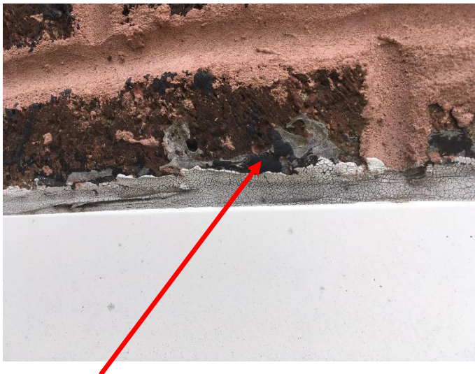
Black tar flashing/sealant
